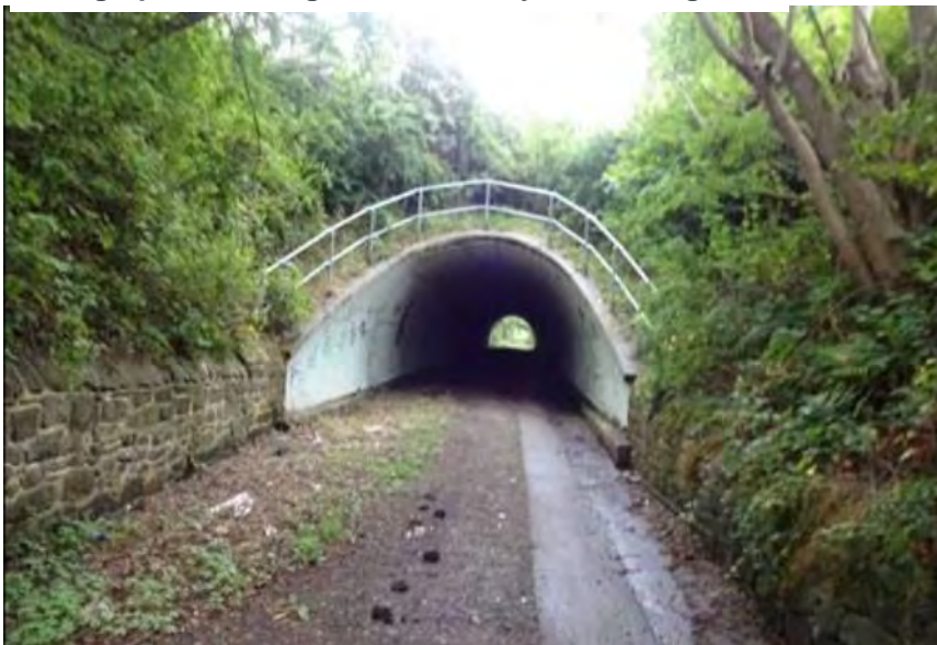
Photograph 6-1 - Longbank Bridleway Underbridge
